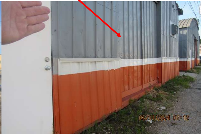
Rear exterior door has been sealed.
